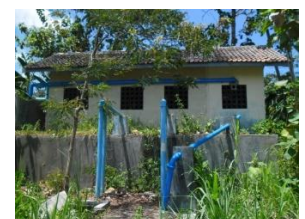
Figure 1. Pump and house of facilities for flowing water from the opak river to the channels
