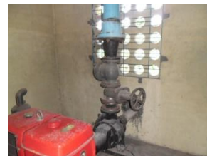
Figure 1. Pump and house of facilities for flowing water from the opak river to the channels
