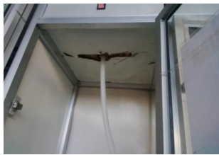
Figure 4. Use of contaminated hoses (Left) and Brittle roof (Right): depots using contaminated hoses. Gallon filling chamber with fragile roof, which causes bacteriological contamination when loading gallons.
