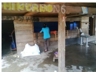
Figure 7. Depot Locations Not Eligible: building conditions are not strong and lighting is not bright enough.
