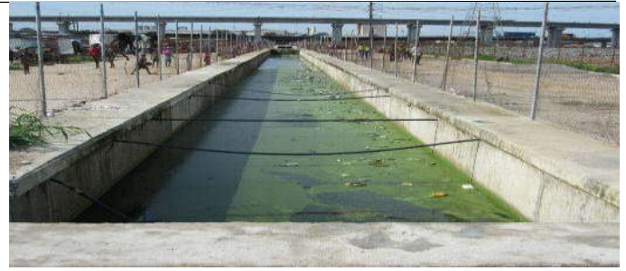
Figure 4. Canal constructed as part of the LMDGP Source: Amnesty International, 2013.
