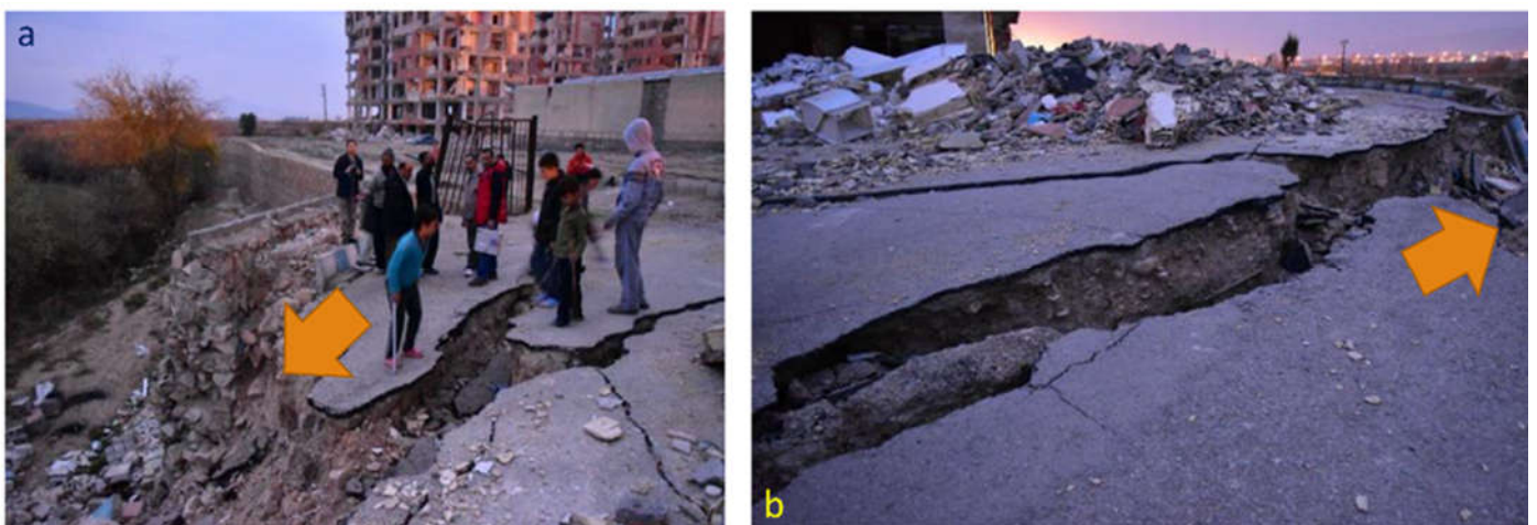
Figure 10. Ground deformation in a) Shahid Shiroodi Mehr housing complex, and b) Foladi District (Miyajima et al. 2018).
