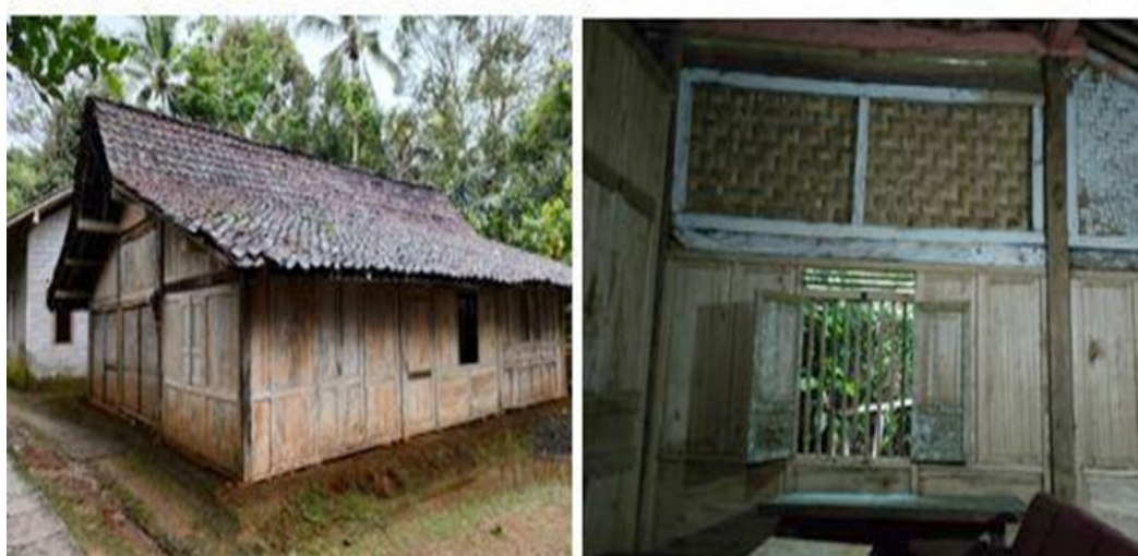
Figure 5. Srotongan Roof Structure: House with Wood and Bamboo Walls
