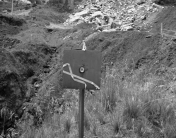
Figure 2: Prism monitoring at the surface subsidence
