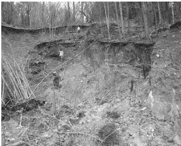
Figure 7: Multi-landslide scars occurred in Western Ranges
