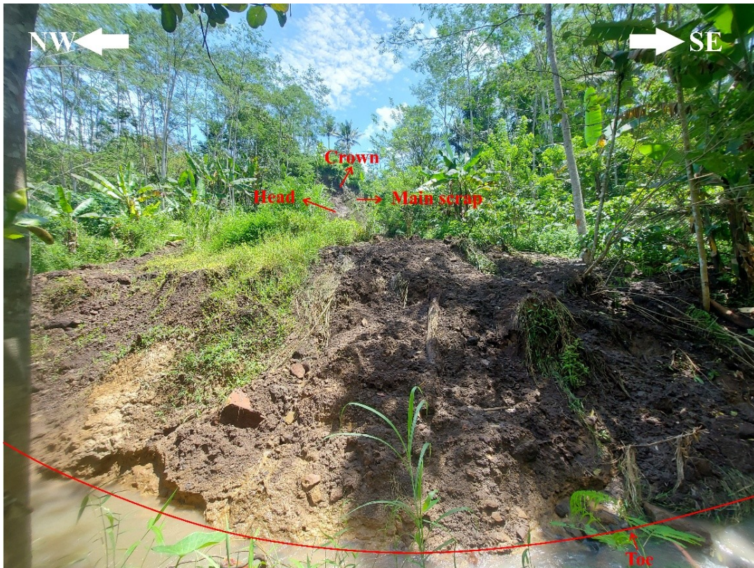
FIGURE 5. Typical landslide observed in the study area.
