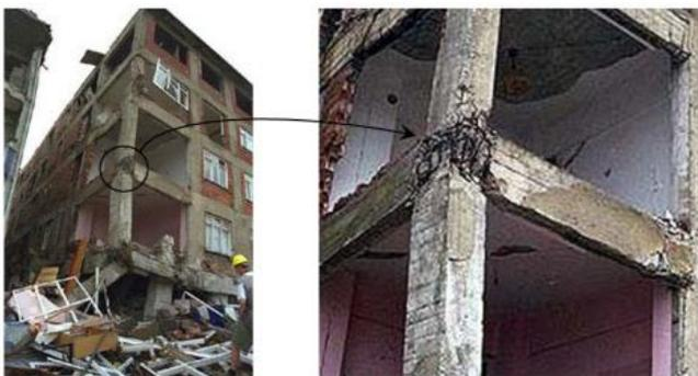
Figure 2. Joint panel damage caused by earthquake (Guner, 2016)
