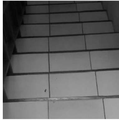
Figure 10. Stair in Water Resources Management Building.
