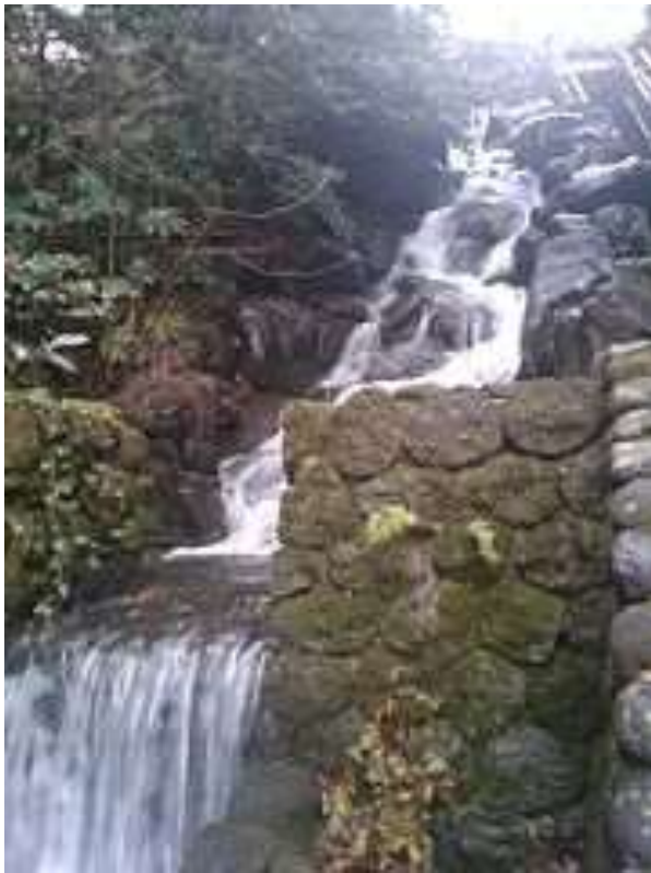
(a). Tatsumi Canal with drop structure ( https://commons.wikimedia.org/wiki/Category:Tatsumi_Canal#/media/File:Tatsumi_canal_(Falls).jpg )
