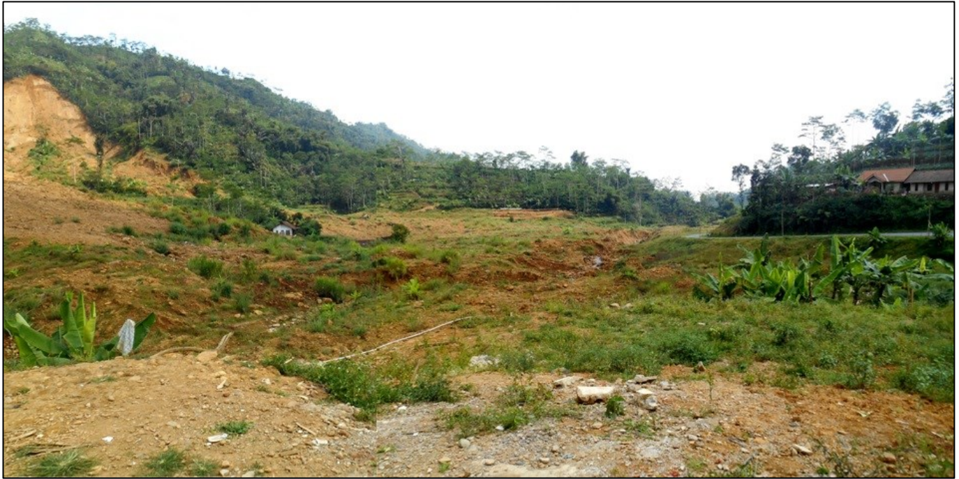
Figure 1. The condition of disaster area after April 2016
