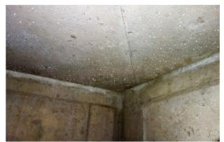
Figure 18. Condensation on the bottom side of the roof slab showing favorable condition for self-healing (Mullem *et al.*, 2020).
