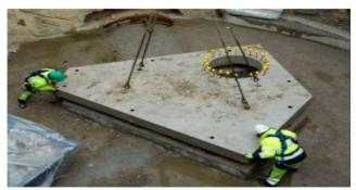
Figure 15. Roof slab made by bio-engineered concrete (Mullem *et al.*, 2020).
