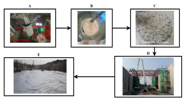
Figure 12. Whole process of the construction of bacteria-based self-healing ship lock wall: (A) Spray drying of bacterial sample, (B) Spore powder, (C) Self-healing concrete mix, (D) Pouring of self-healing concrete, (E) Curing of self-healing concrete (Zhang and Qian, 2020).
