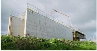
Figure 10. Full scale demonstrator nn situ cast self-healing concrete water reservoir (Mors & Jonkers, 2019).
