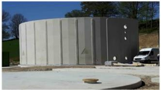
Figure 9. Prefabricated wastewater treatment tank by using self-healing concrete (under construction) (Mors & Jonkers, 2019).
