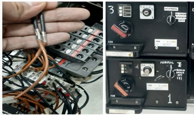
Figure 7. On/Off Switch Modification Result
