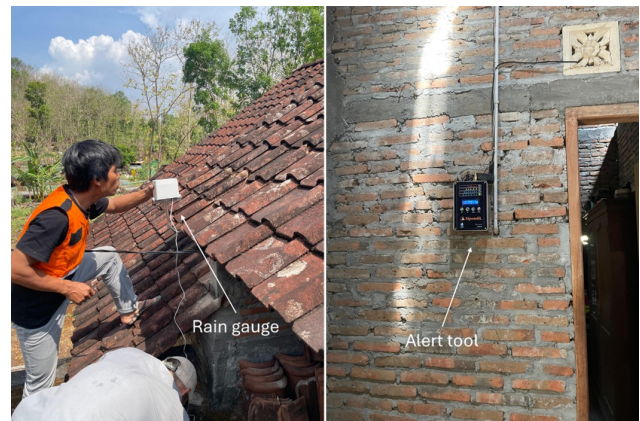
Figure 8 . Community-based installation of Sipendil. Sipendil is a rainfall-threshold landslide early warning system based on rainfall scenarios
