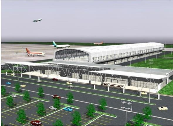
Another significant change from previously existed terminals is the use of glass as building's side wall. Usage of glass also made the efficiency on electricity spending by day because of natural sunlight that goes straight into the building so the usage of lamps can be reduced. There is also change saw on the colour palette usage, which is dominant turquoise for the walls and yellow for the signage, marking the modern era of simple and functional building.
