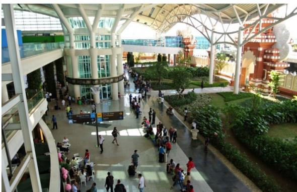
The roofing structure for the upper floor is tilted flat roof that sustained by tilted concrete post and steel frames and then enveloped by aluminum cladding. Details were not much seen but it saw some advancement by adding the wood material on wall
