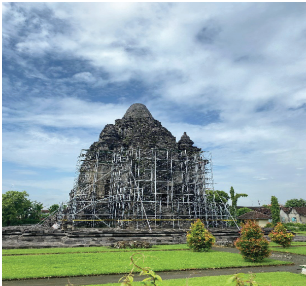
Figure 1. Restoration of Kalasan Temple in progress
