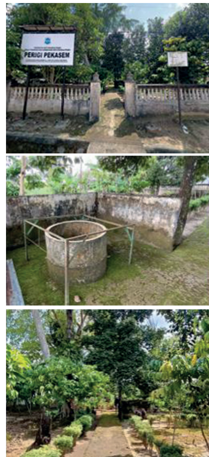
Figure 5. Condition of Perigi Pekasem. Front facade of Perigi Pekasem (left), Heritage structure of Perigi Pekasem (middle), and the garden area inside the site (right). Source: Author's documentation (2022).
