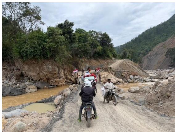
Figure 1. Collapsed Bridge Infrastructure Limiting Access to Health Facilities in Disaster-Affected Highland Areas of Bener Meriah Regency.
