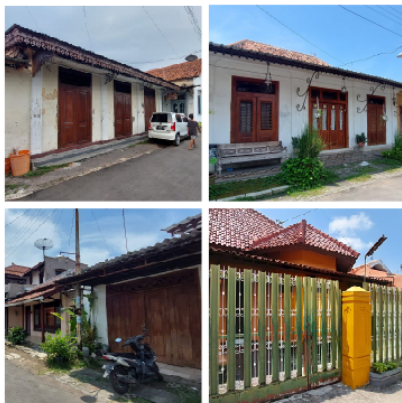
Figure 7 Old Heritage Building in Zone A
