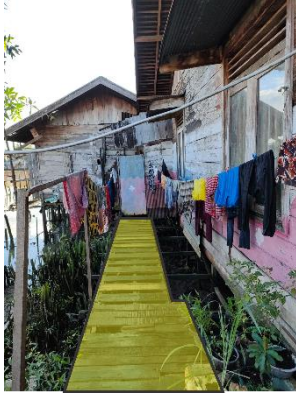
Figure 19. Batang with Stilt Structure Source: Author (2022)
