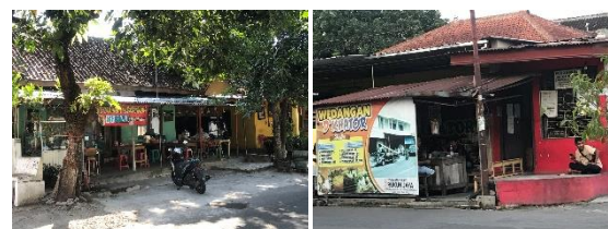
Figure 2. The Condition of Kampung Karengan
