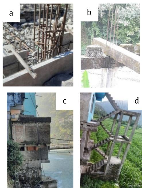
Figure 5 (a) No proper anchorage in column-beam joints and stirrup spacing (b), (c), and (d) poor column-beam joint spacing.
