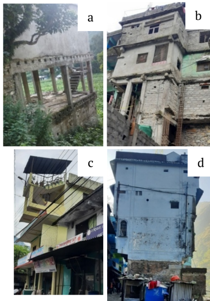
Figure 6 (a) Poor column-beam joints, a soft story; (b) poor beam column, soft story, floating columns; (c) Load accumulation in the upper floor; (d) floating columns.
