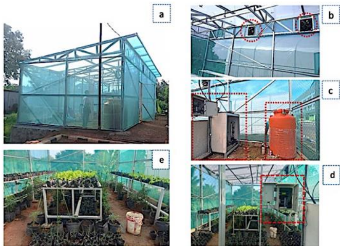
Figure 8. Smart greenhouse and control system: (a) exterior structure of the smart greenhouse, (b) roof-mounted automatic circulation fans, (c) water tank and pumping system for irrigation, (d) control panel with electronic devices, (e) plant cultivation area inside the greenhouse.
