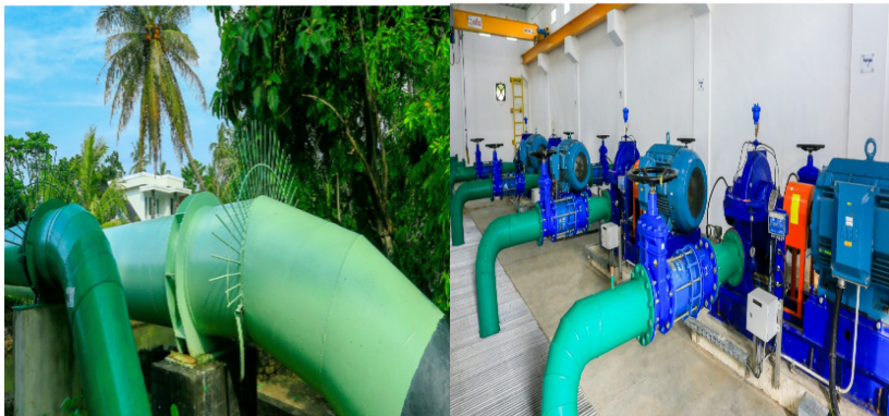
Figure 3. Diameter Transmitter Pipe Line (1.4 metres) and Pump House (Pump Station)
