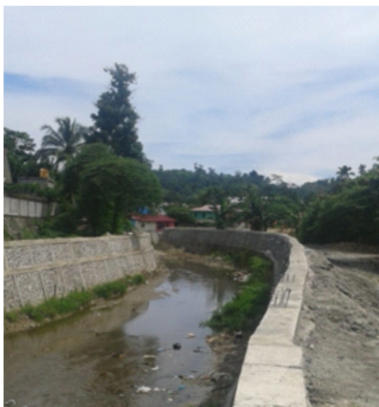
Gambar 2. Tanggul telah selesai Figure 2. The embankment has been finished
