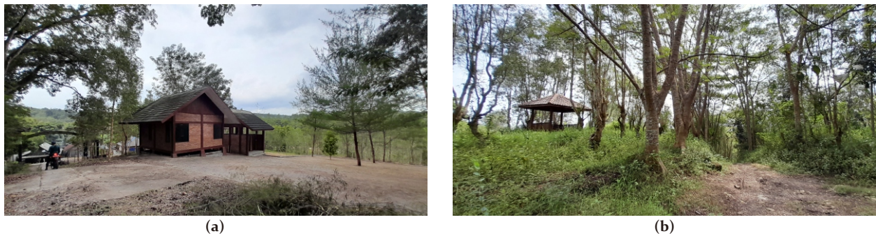
Figure 14. The facilities and infrastructures in the form of a work hut and toilet in the utilization block of plot 15 (a) and a monitoring gazebo in the protection block of plot 21 (b)
